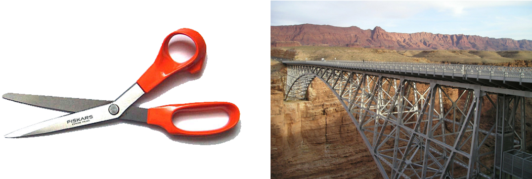
Figure 6.1.1 Scissors and bridges are examples of engineering structures. Scissors are machines with three interconnected parts. The bridge is a truss.
